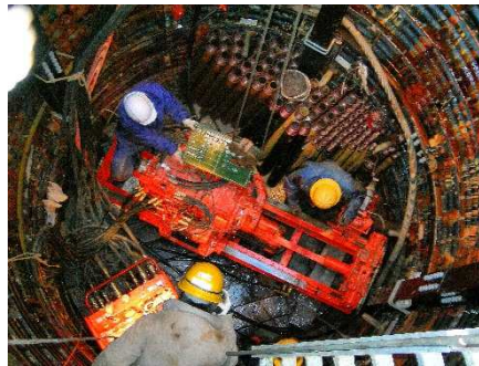
Dewatering hole drilling inside manhole
