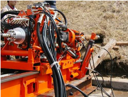
Dewatering hole drilling
