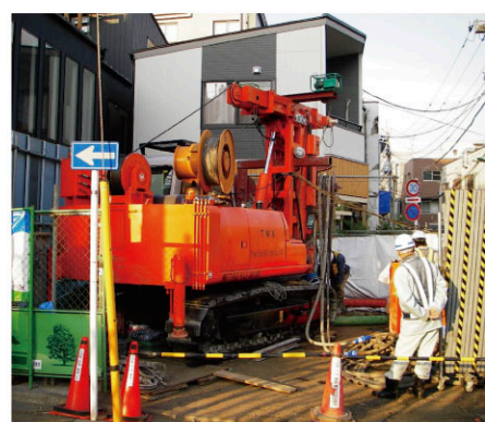
鉄道地下化(TMX) Diaphragm wall construction for underground railway station
