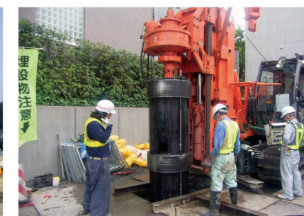
既設鋼管杭の撤去 Removal of existing steel pile
