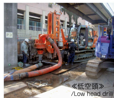
《低空頭》 /Low head drill 橋梁下(MPD) Foundation piling under flyover
